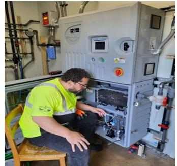
Maintenance Worker 3, Scott Newton, is seen monitoring water system conditions with our telemetry system, which requires 24-7 monitoring and daily documentation for compliance to ensure safe drinking water and good system operation.
