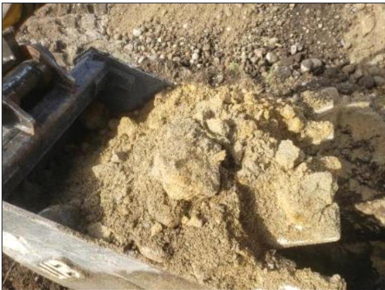
**Photos GTP-102:** Test Pit GTP-102 to approximately 8½ feet in depth (below); Sample from bottom of exploration at 8½ feet (left)
